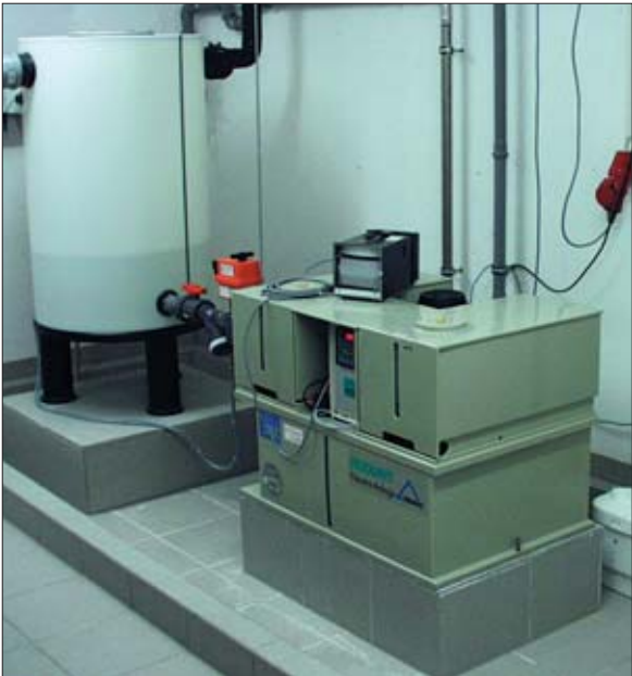
Built-in example FRIDURIT® neutraliser unit with storage tank
