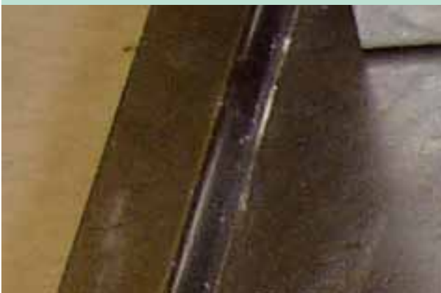
Laboratory benchtop with bonded marine edge
