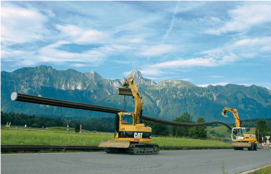
■ Excavators transported the pre-fused pipe sections to the place of installation
