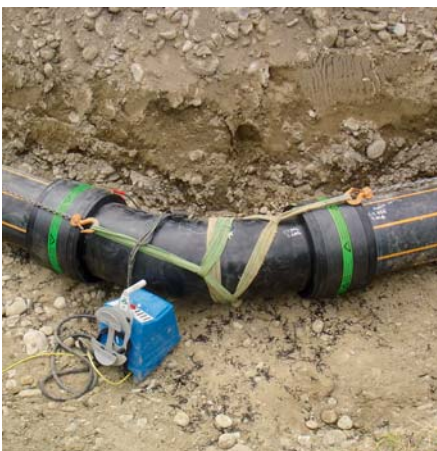
■ The PE elbows were fused using a FRIAMAT fusion unit
