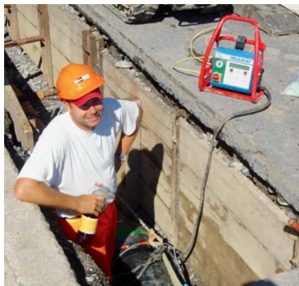
■ The PE fittings were fused using a FRIAMAT fusion unit
