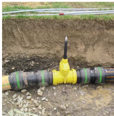
■ A shut-off valve integrated with FRIALEN Safety Fittings
