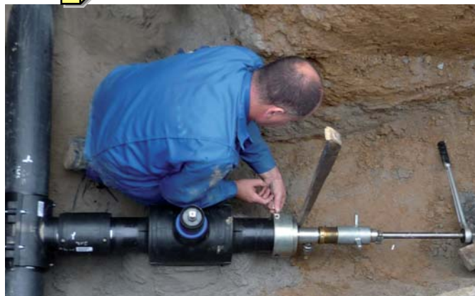
Picture 3: Drilling via standard flange, valve and SAFL
