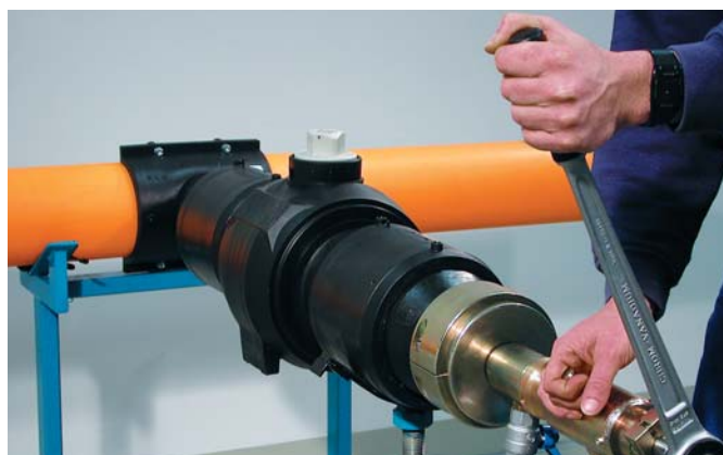
Picture 4: Drilling via clamping fixture and ball valve
