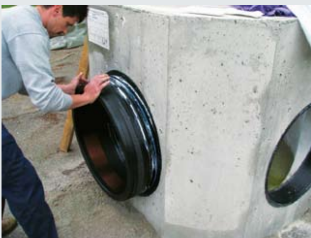
FIG. 11: Connection of PE pipes to a concrete manhole base with sewage inspection chamber adapter ASF and insert sleeve AEM
