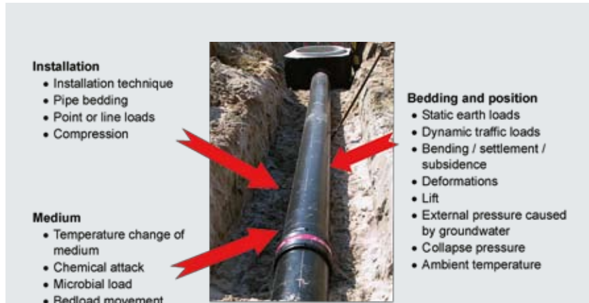
FIG. 1: Load types of a sewer piping system
