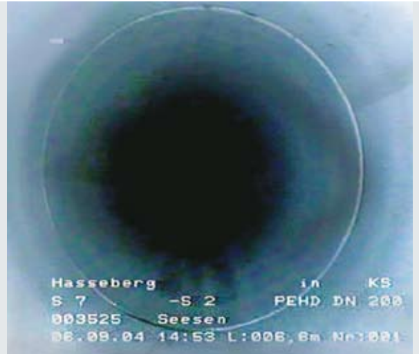
FIG. 5: Reality: Camera inspection of the sewer: hydraulically smooth pipe joint
