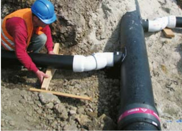
FIG. 13: Domestic sewer pipes are connected using the sewage saddle ASA-TL, in this case in connection with sewage bends ABMS d 160mm
