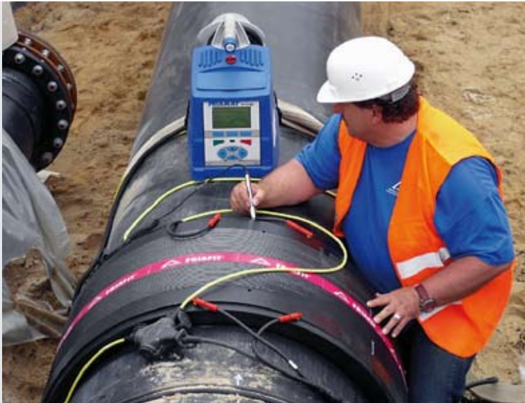
FIG. 6: PE pipe, joining method: electrofusion technology, coupler and electrofusion unit
